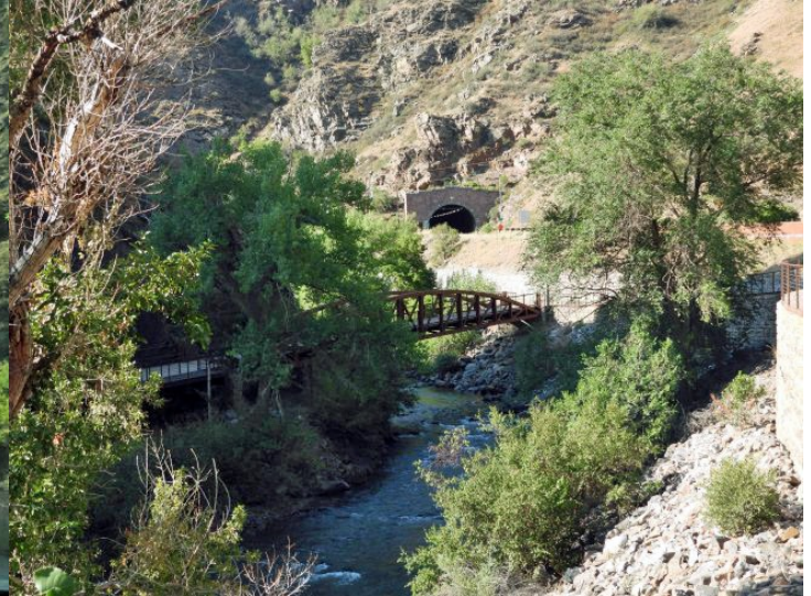
Road tunnel #1 is beyond the trail bridge above Clear Creek.
