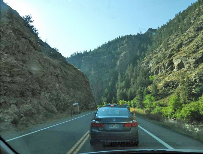
Daily construction made everyone stop to take turns on a temporary one-lane road section about a mile long.
