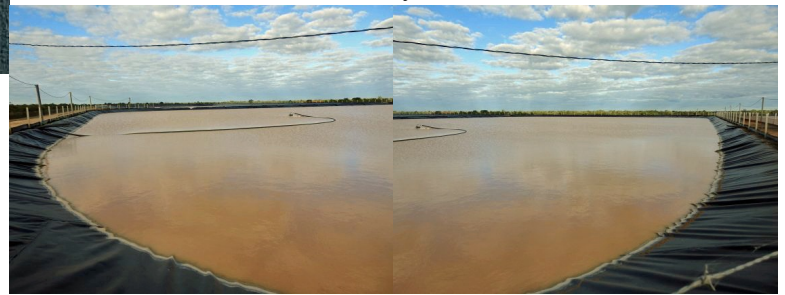
Lined water collection pond
