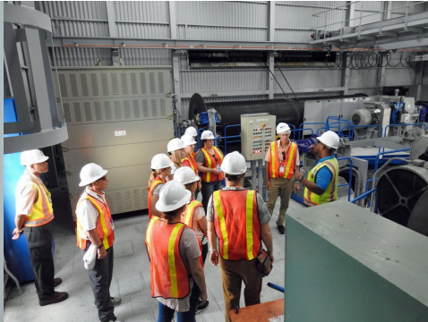
Arrival in room with motors and cables.
