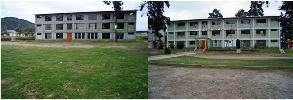
Second school building, being finished. First school building.
