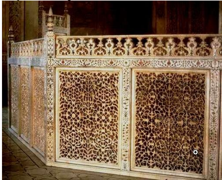
Lattice of carved marble, allowing viewing through it.
