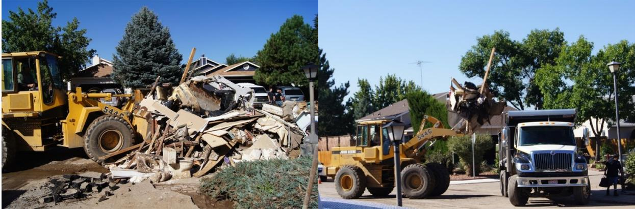
Large front-end loaders were needed to remove the piles of trash, assisted by a smaller Bobcat (its white arms showing above the trash) pushing the debris into the bucket of the larger machine. Large trucks then were filled with the debris and carried it away to some landfill site.
