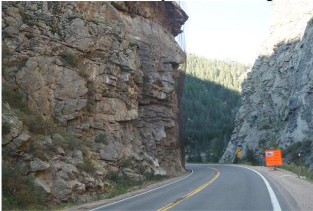
The first photo is of a narrow passageway in Clear Creek Canyon. In the center the cliff is covered with a rusty wire mesh to reduce the falling of rocks onto the highway.
