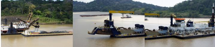
The canal is being dredged to make room for larger ships. Some equipment loads debris onto barges, as at the left. Other equipment continuously digs sediments and pumps them to the shore using large pipes, such as those rafted in the background of the middle photo. Several times we saw trains on the east side of the canal carrying containers between the port cities. The white tower behind has ship navigation aids.
