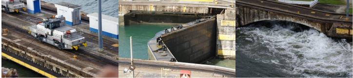
Electric powered tractors on both sides of the ship use tight cables to keep the ship centered in the locks and away from its walls. The tractors do not pull the ship, which moves under its own power. The lock doors in the center photo are closed shut while the water on its left side drains. The right photo shows turbulent water that has drained from that lock. All water eventually goes into the ocean.
