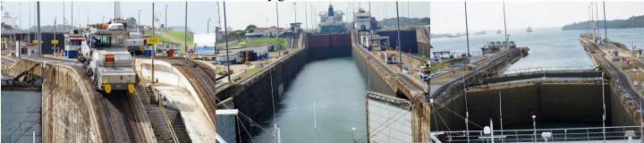
The left photo shows a tractor climbing up an incline using the ladder-like track under the tractor. The center photo shows us about to enter the middle lock. The upper right photo shows us in the last lock before being raised to the level of the lake beyond. The lower right photo shows the tight clearance for the container ship, which has the maximum width allowed by the canal. It illustrates the need for the wider locks that are bring constructed nearby.
