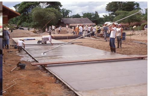
Smoothing the concrete
