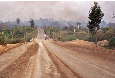
Smoke ahead. Fixing of the road.
