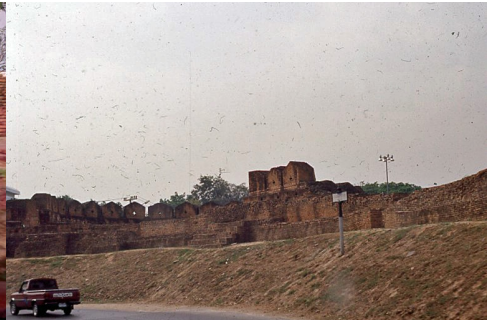
Some large wall structures
