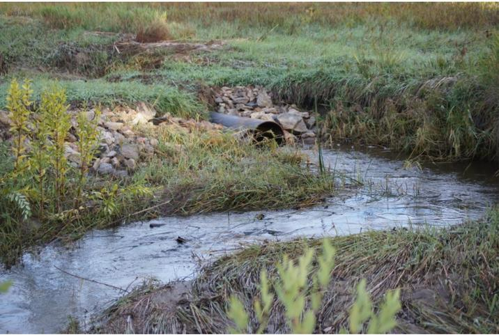
84. Receding water, 7:50 AM, 29 September 2013, revealing some scouring above culvert.
