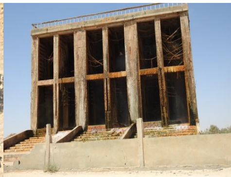
Tower for spraying the hot water for initial cooling.
