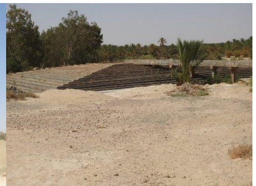
Spiral pyramid for further cooling of the hot water.
