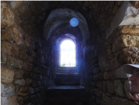
Exit stairs and door (locked gate).
