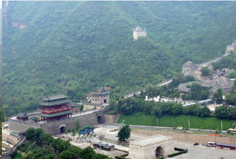
A view of the south part of the loop.
