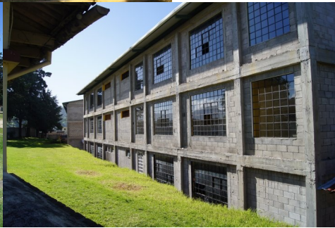
The newer school building being fixed.
