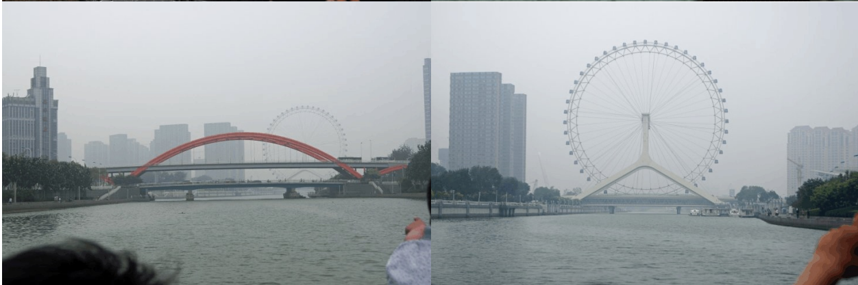
A double deck bridge.
