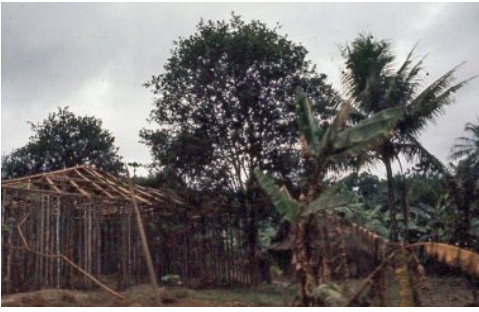
House frame ready for mud throwing
